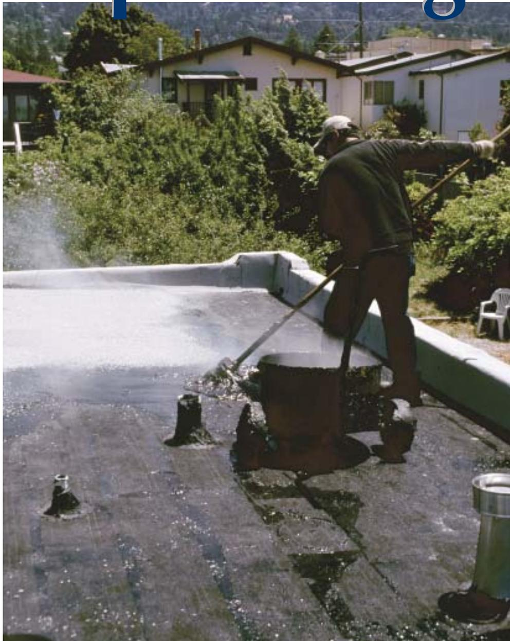
**Figure 1.** BUR is applied over wood, concrete, steel, or foam insulation. The original part of this house has one-by board sheathing, but the addition has plywood. Either substrate is fine, as long as it's structurally sound and solidly fastened.
