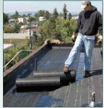
**Figure 11.** The roofers apply successive layers of felt over hot asphalt. On this roof, full sheets lap  $\frac{2}{3}$  onto the sheets below, which means there will be at least three layers of felt plus one layer of base sheet at any given point.
